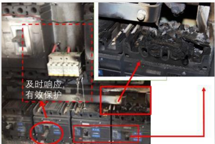
DC disconnector broken
