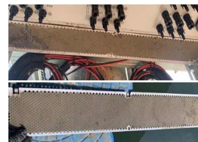
Ventilation Panel blocked by dust
